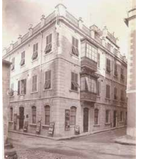
The original facade of Cloister Building.
